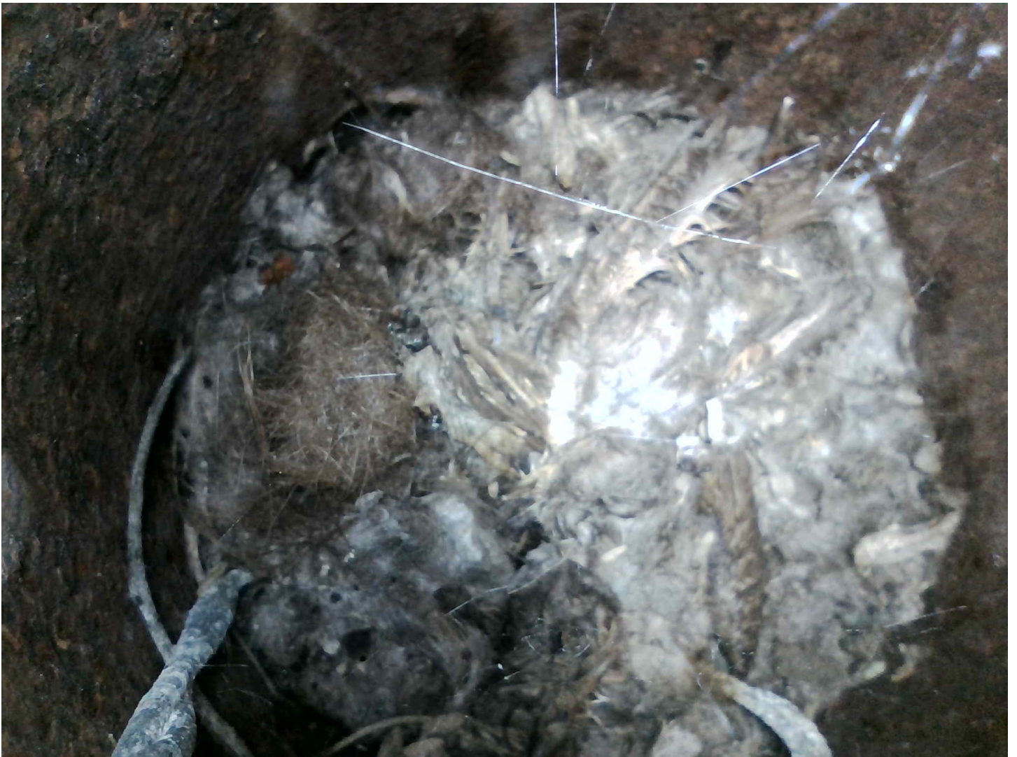
Figure 4 Remains inside of an open pipe: fur, feathers and bones of perished animals.
