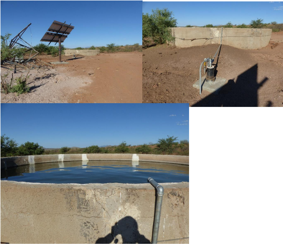
Soapweed Well and Existing storage
