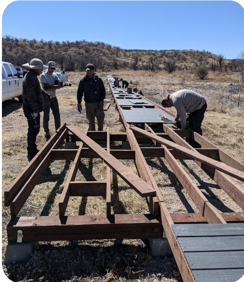
Installing the boardwalk at Arivaca Cienega. The wide spots for are pull outs to admire the view without stopping other traffic.
