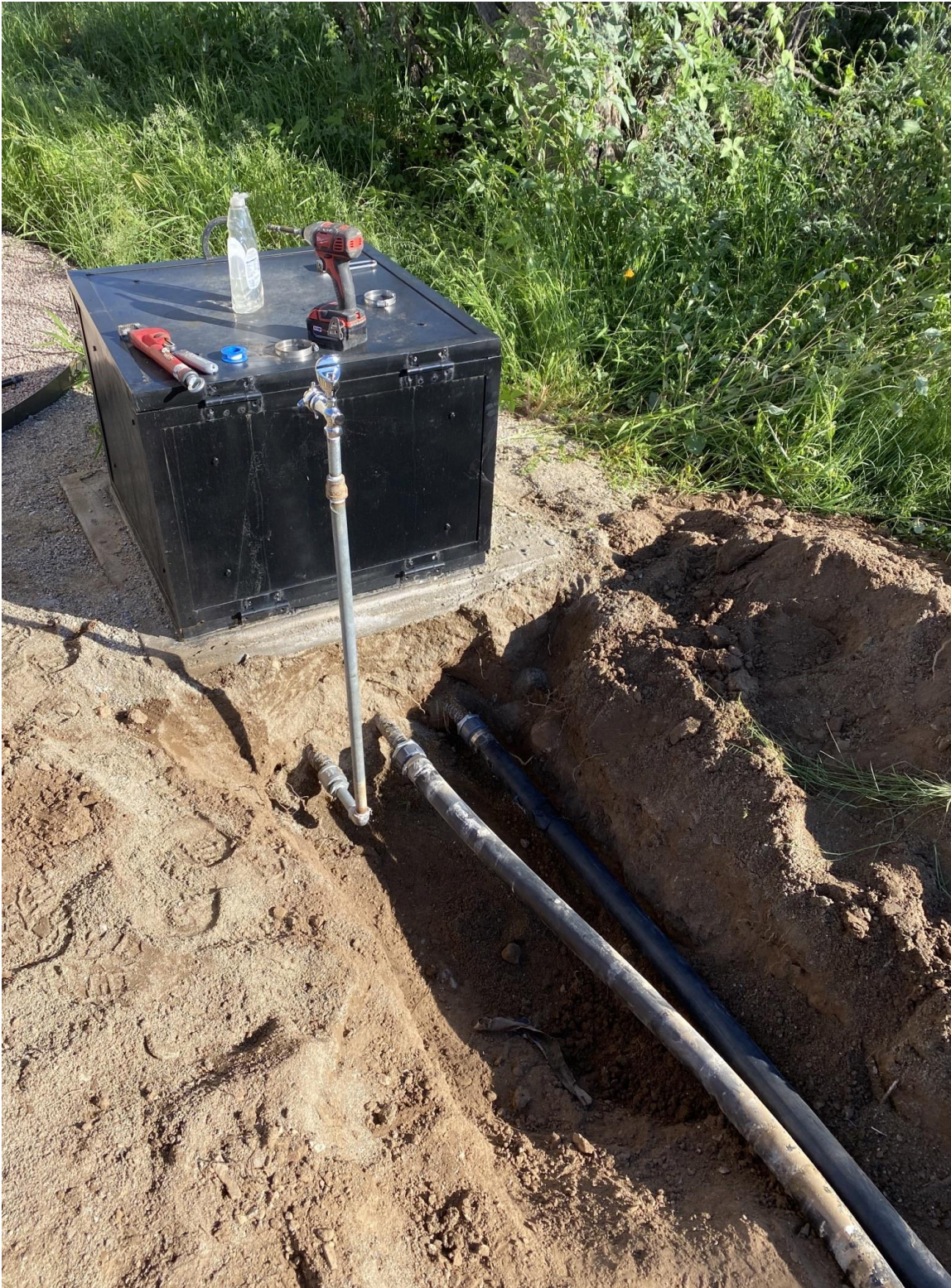
Two levy lines installed into gate valves
