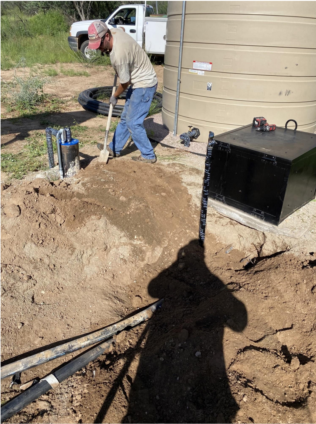
Making connections to the well head
