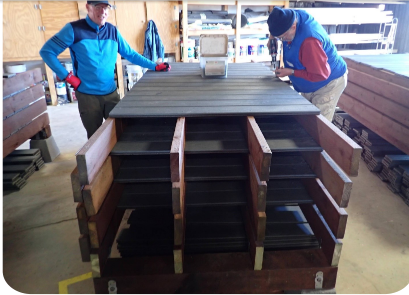
Stacks of boardwalk constructed by volunteers in the refuge carpentry shop.
