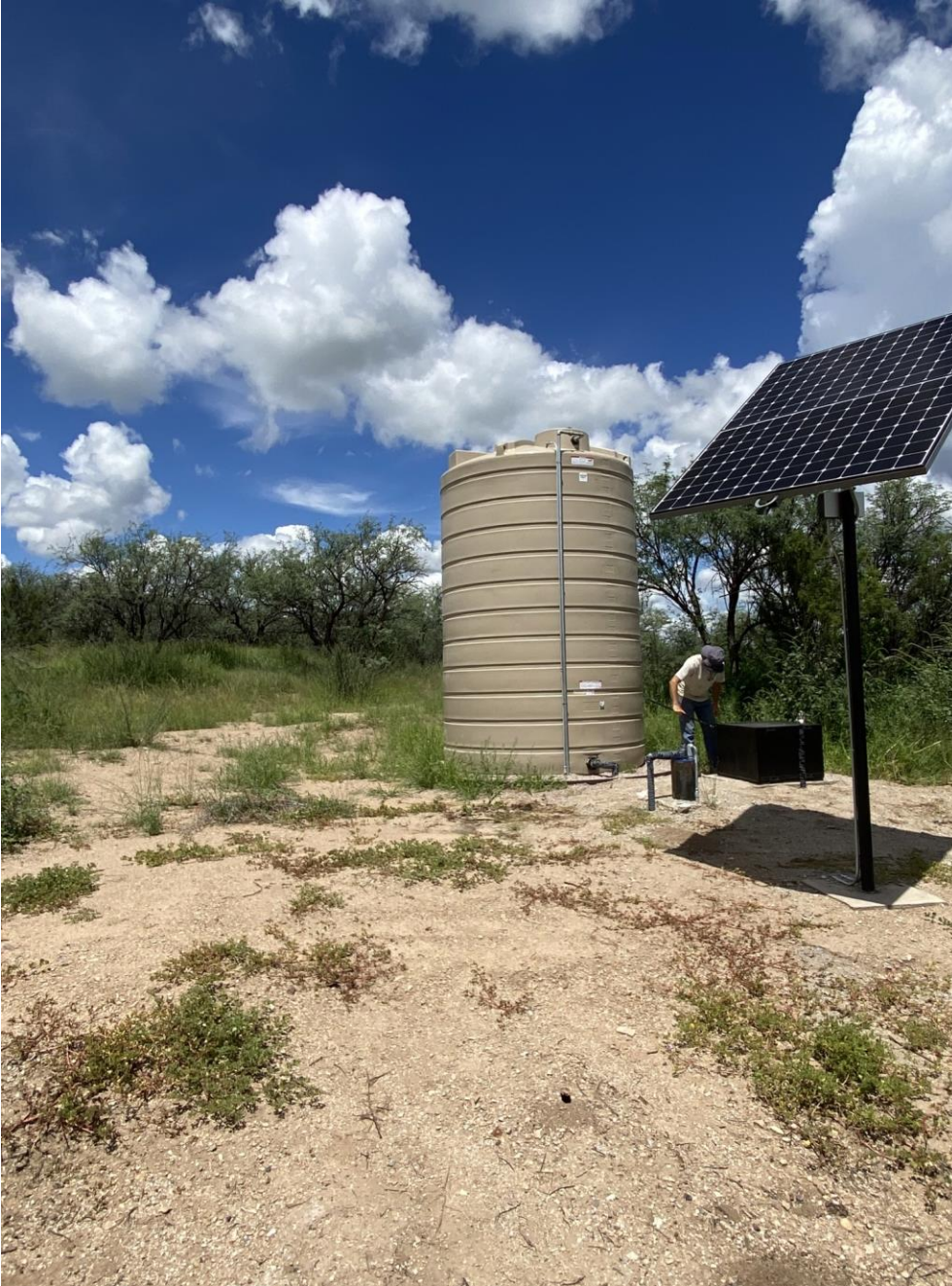
5000 gallon poly tank, solar panels and solar pump and motor
