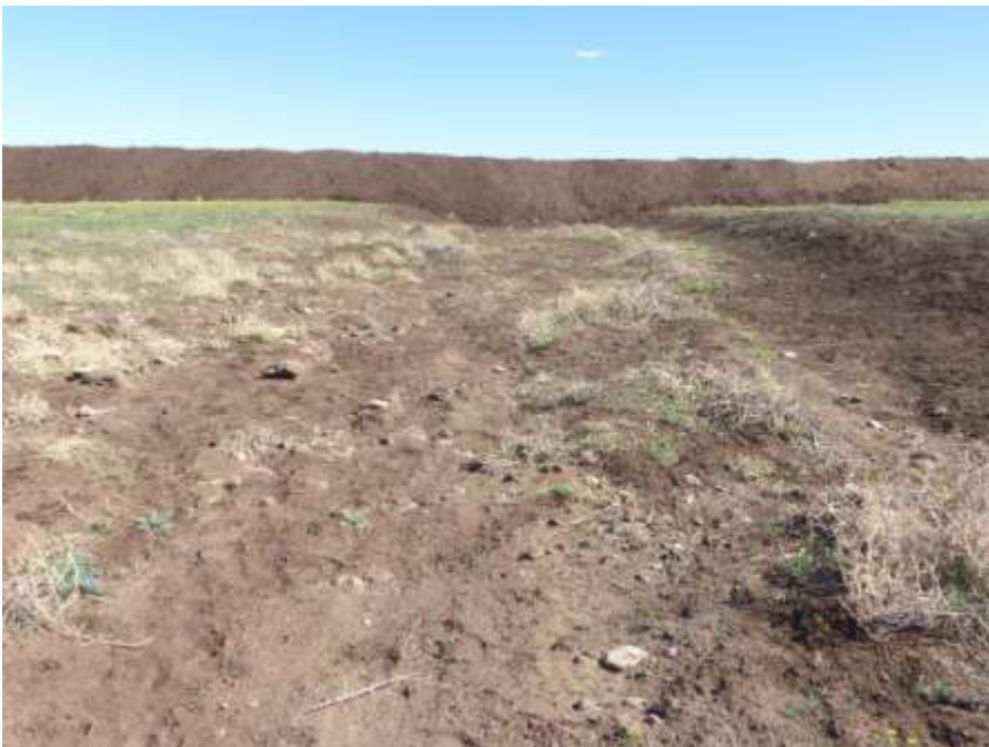
Downstream view of repaired dam
