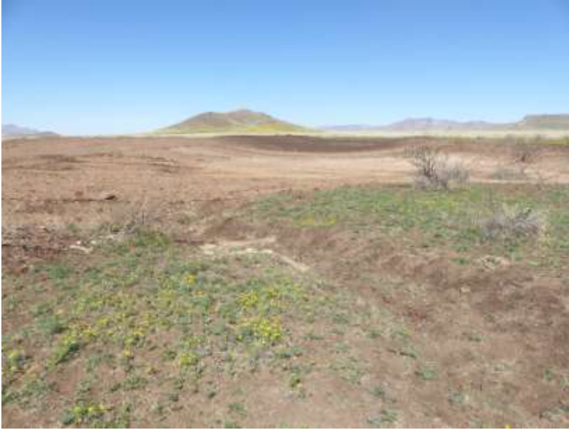
Overview of Back Pasture Tank repair
